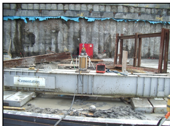
Plate 8: Tension test reaction system at Spencer Dock
