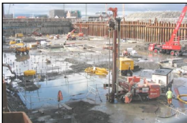
Plate 7: Drilling for bar anchors at Spencer Dock using DTHH techniques
