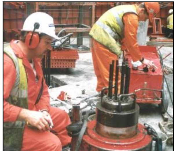
Plate 3 –Stressing of Tendon Anchor
