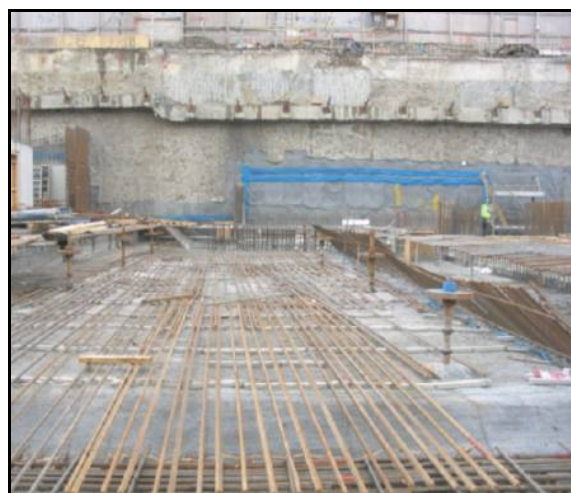
Plate 6: Bar anchors with head plates fitted and slab reinforcement being fixed
