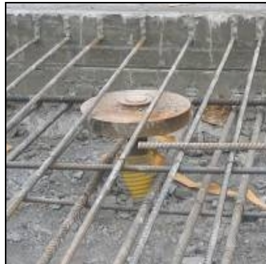
Plate 4 – ATM head plate prior to casting of basement slab
